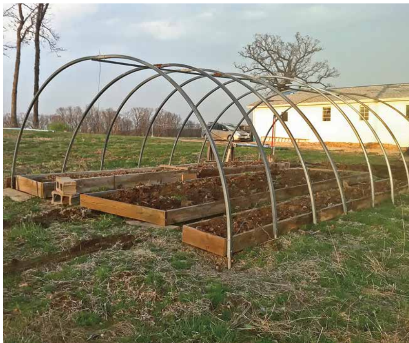
FIGURE 1.6. I used square steel tubing to build my hoop house in Missouri, which I used to grow year-round for many years. I placed smaller hoop houses over the raised beds to create a warmer microclimate, allowing me to grow cold-footed veggies throughout the coldest of winters.
