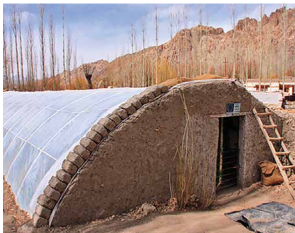
FIGURE 1.9. Chinese greenhouse. The greenhouse shown in the photo is earth-sheltered on the north side. Also note that there is no glazing (glass or plastic) on the east side. Compare it to the above-ground greenhouse shown in Figure 1.8. Courtesy of Dr. Sanjun Gu.
