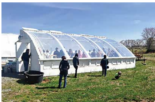
FIGURE 1.8. An above-ground (Americanized) Chinese greenhouse in southern Tennessee. Don't be deceived by this design. True Chinese greenhouses are earth-sheltered to permit wintertime production without costly fossil fuels. I'd be very leery about above-ground constructions. I'll explain why in the next chapter.
