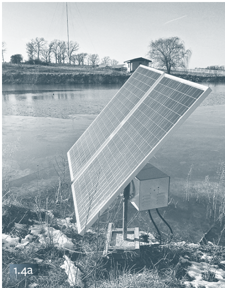
Figure 1.4. (a) Aerating my half-acre farm pond reduces bottom sludge and helps create a healthier environment for the fish. (b) To prevent the pond from icing over completely in the winter (so our ducks can swim), I designed and installed a solar pond aerator in conjunction with a St. Louis company, Outdoor Water Solutions. They are currently selling a design like this online. Credit: Dan Chiras.
