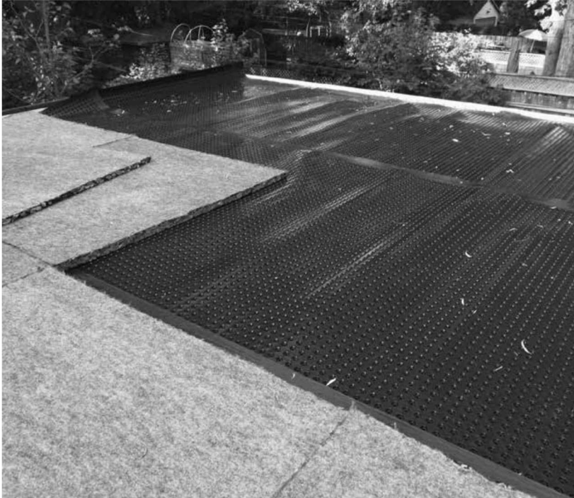
Fig. 1.3: A built-in-place system is installed in layers on the roof.
