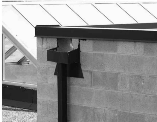
Fig. 2.5: A flat roof with a typical scupper. Scupper openings allow for water to exit the roof and into a downspout.
