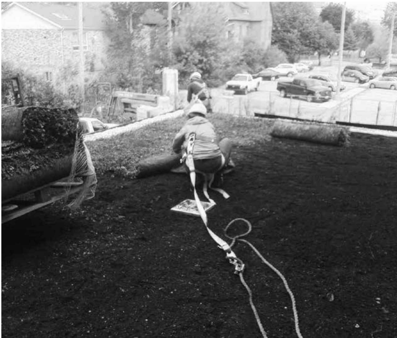
Fig. 1.4: An example of a hybrid system: layers are installed individually and finished with pre-grown vegetation mats. PHOTO CREDIT: RESTORATION GARDENS, INC.
