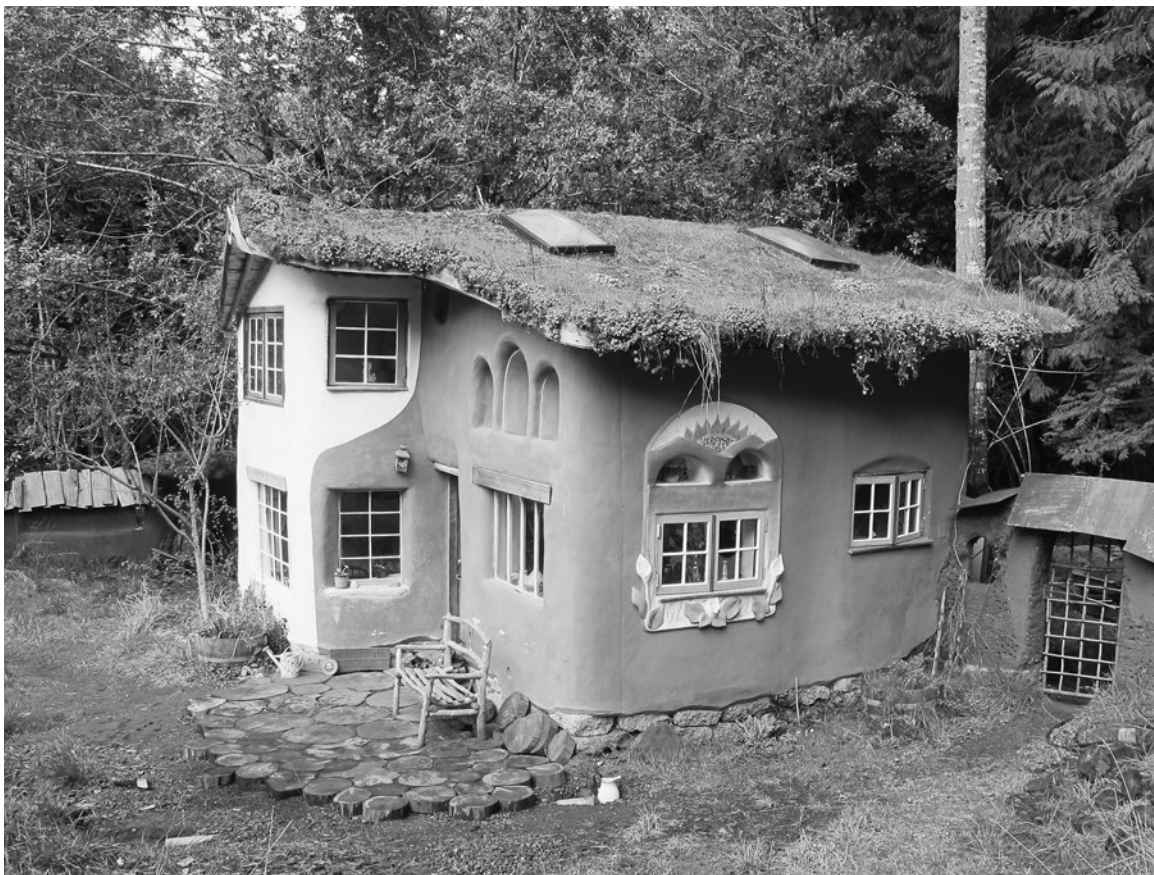
“The Laughing House” at Cob Cottage Company headquarters in the Oregon rainforest is a typical example of Oregon Cob: small, highly sculptural, and constructed largely of site-harvested and salvaged materials. CREDIT: MICHAEL G. SMITH
