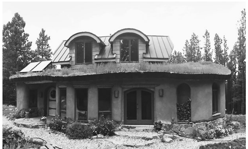
Cob lends itself to curvilinear forms and whimsical designs. Kindra Welch designed this mountain retreat for family members in northern New Mexico. The cob walls were built primarily in work parties by previously untrained volunteers. CREDIT: CLAY SAND STRAW
