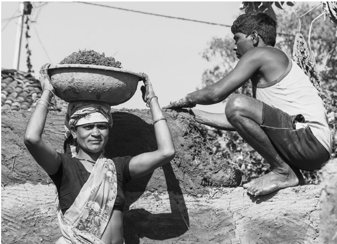
Villagers in the Indian state of Punjab building a cob house in 2020. This is one of many parts of the world where ancient earth-building traditions have been passed down generation to generation to the present day. CREDIT: SANSKAR HARDAHA/ALAMY STOCK PHOTO
