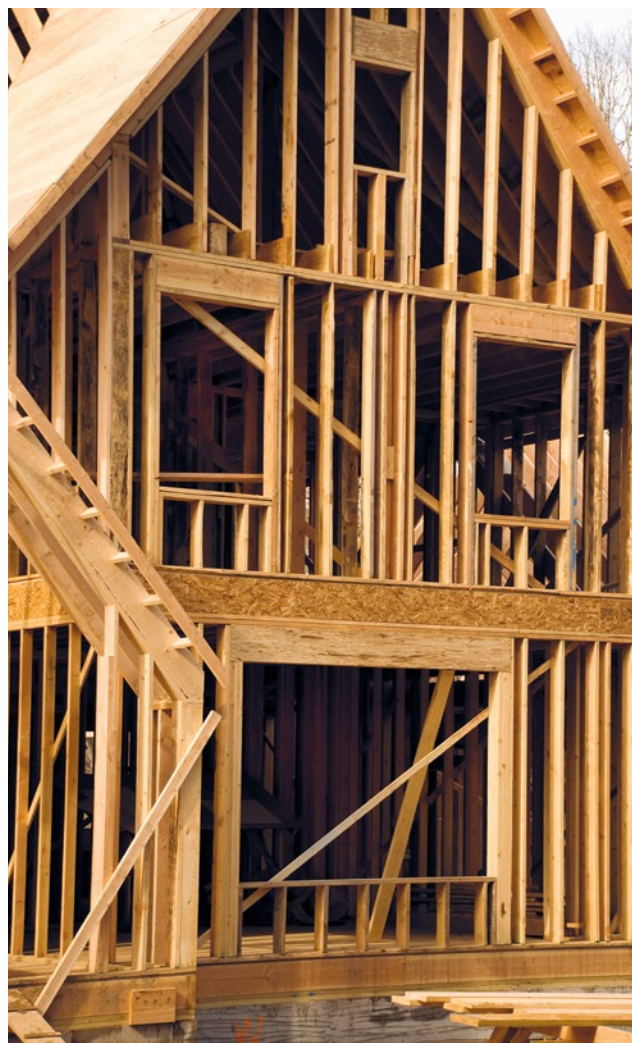
Wooden stud framing in progress.
