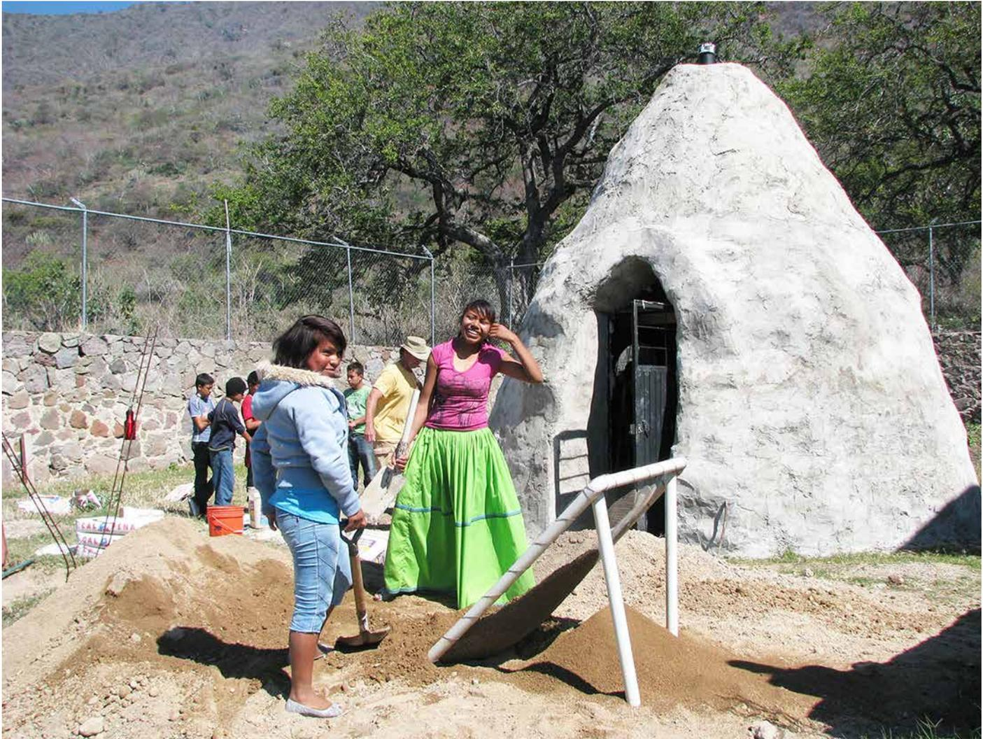
**Fig. 3.1:** This small earthbag dome under construction in Mexico was plastered on the exterior with cement-based stucco that had a latex additive to make it more waterproof. In addition, it was painted with a couple of coats of water-impermeable roof paint. CREDIT: KELLY HART
